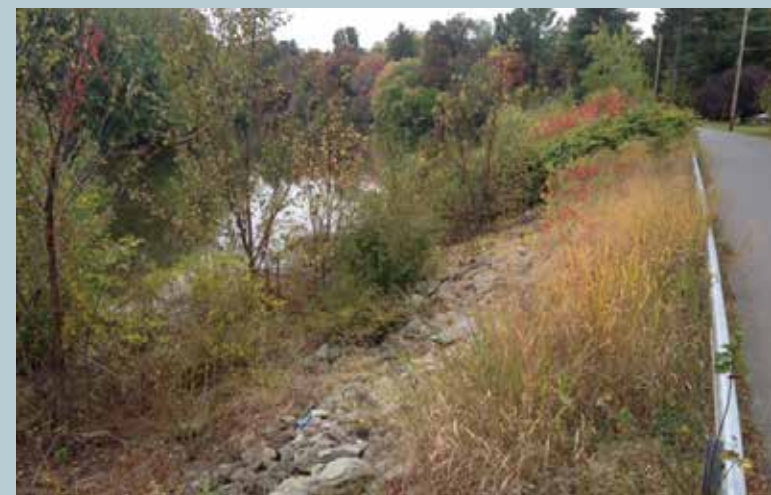
Living shoreline constructed by ACOE on the Wallkill River in Rosendale, NY - mix of boulders and vegetation.
